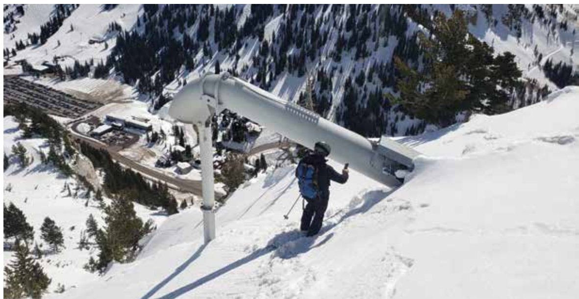
A Gazex 1.5 used by the Utah Department of Transportation above Highway 210 in Little Cottonwood Canyon, Utah. The Alta Ski Area parking lot is visible to the left.
