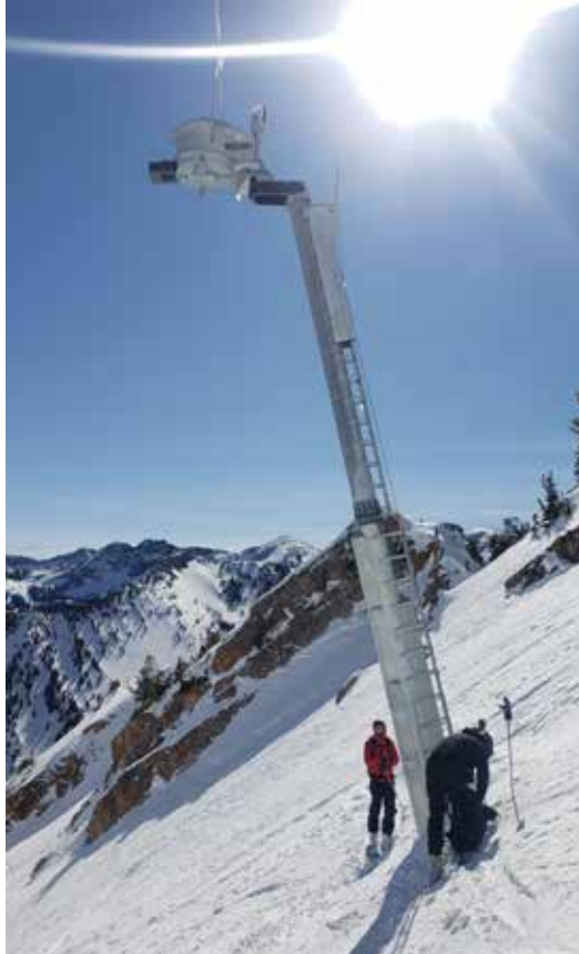
Wyssen Tower system in Cardiff Bowl, Little Cottonwood Canyon, Utah.
